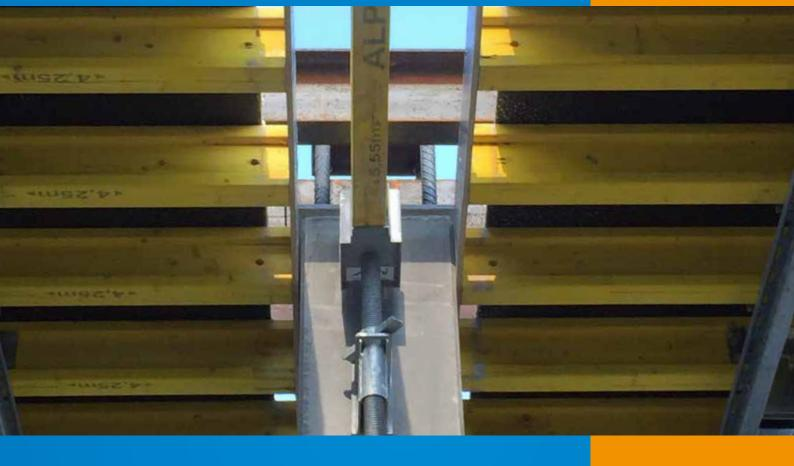
This support bracket can be used with all commercially available beams compatible with the two-inlet fork. It can be mounted easily, on a skin, post or girder, using a concrete screw.
